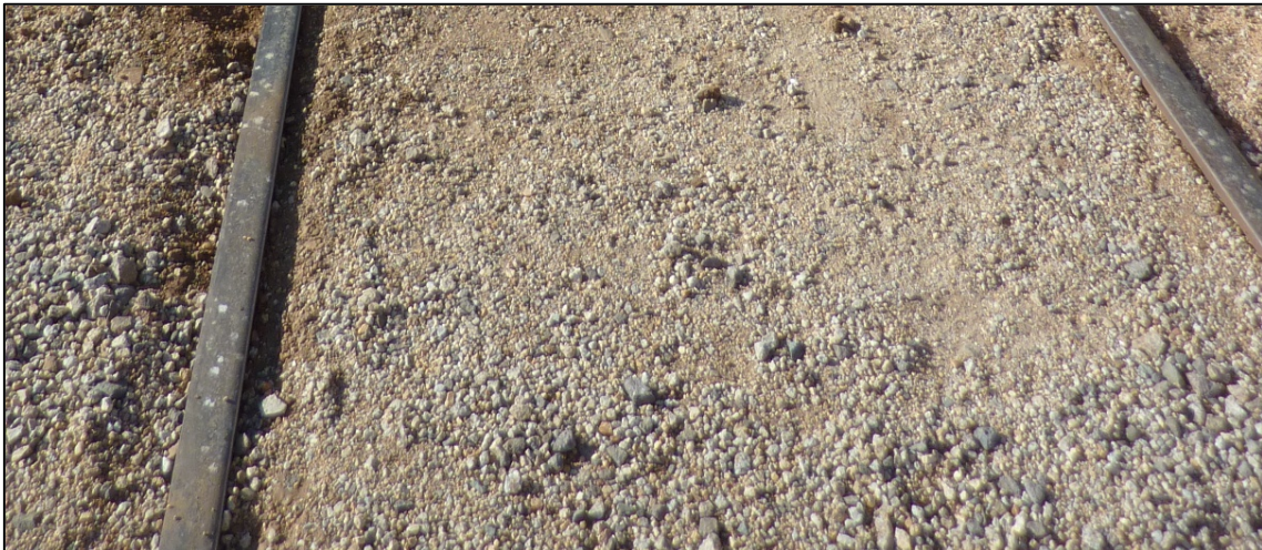
Figure 5: Level crossing surface and buried rail
