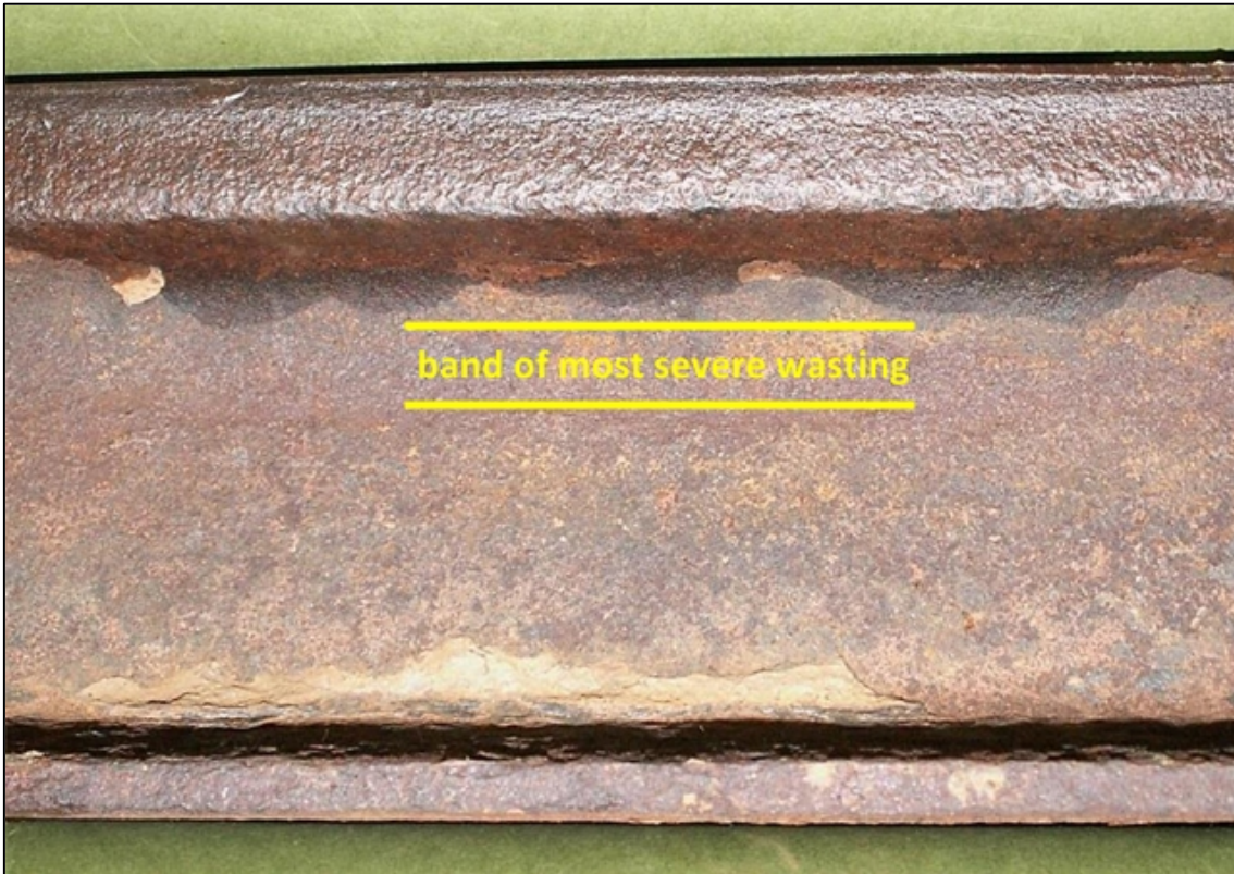
Figure 15: Corrosion band on intact rail
