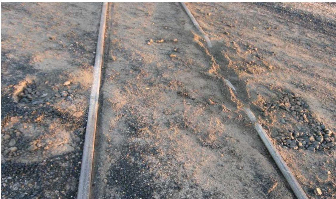
Figure 13: Mellis Road level crossing, Warracknabeal
